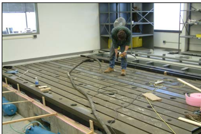
Grouting using grout holes.
