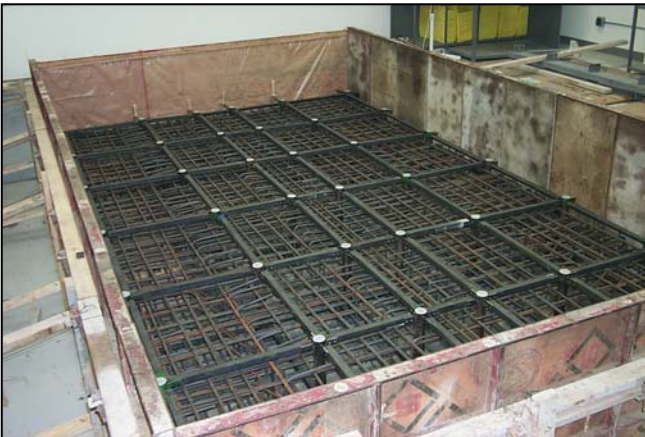
Form work, rebar and anchor frame installed
