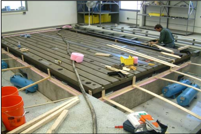
Preparation for grouting the plates.
