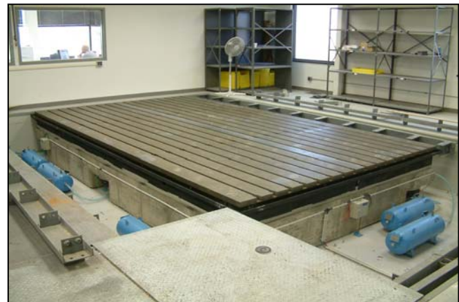
Finished: Protective wax on the plate stays until all subcontractors finish the work and test system is ready to be installed.
