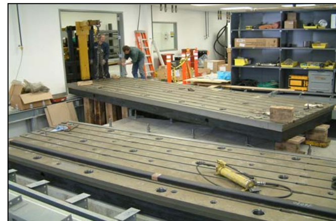
Bringing in the second sub-plate and connect sub-plates via high-strength bolts to form larger plate area.
