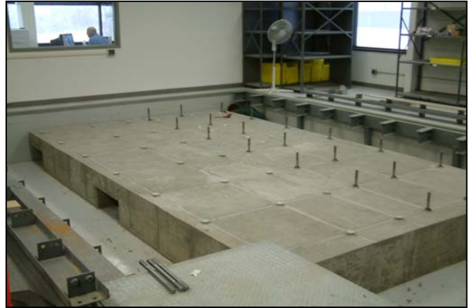
Installed anchors for first STOLLE sub-plate
