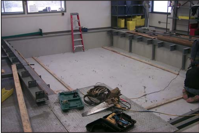
Seismic Mass area
