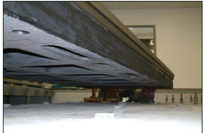
Moving plate into location. Plate bottom with ribs and machined drip edge for fluid trough visible.
