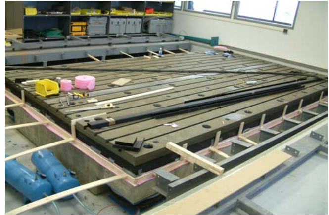
All gaps are framed and plate is ready for grouting.
