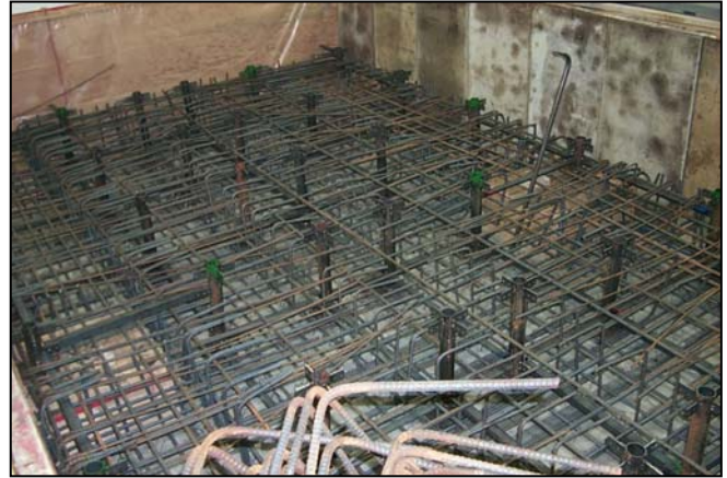
Rebar with anchor frame, upper connecting bars not installed yet.
