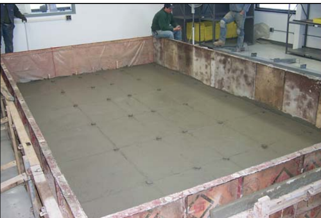
Finished seismic mass
