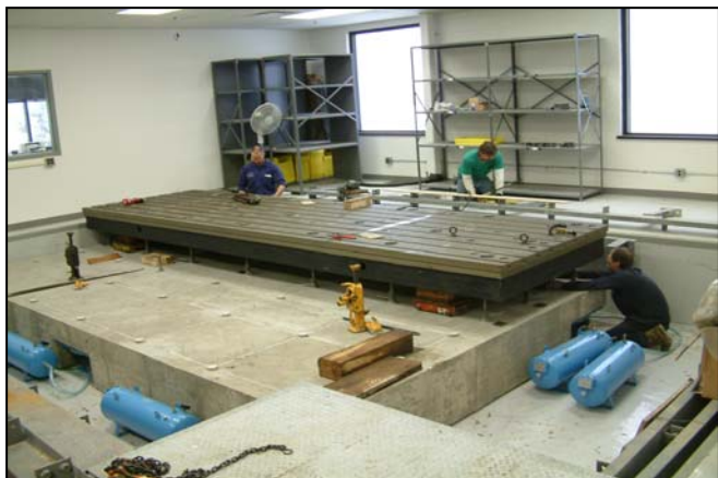
Adjust and level first sub-plate
