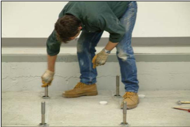
Inserting the anchors into the anchor frame
